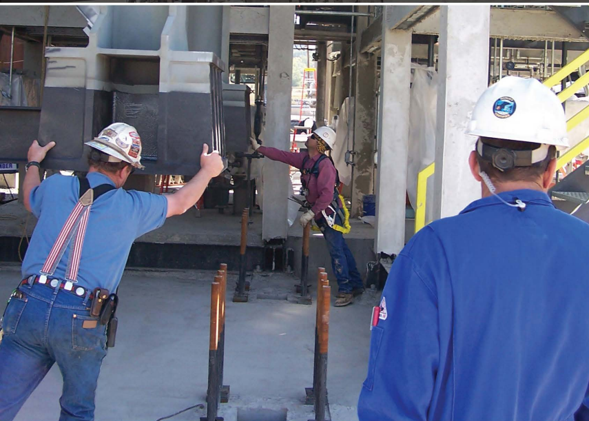
Installation of Support System - Cycle X - Flying J
