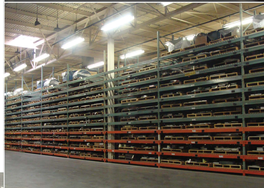
Narrow Opening Rack Storage
